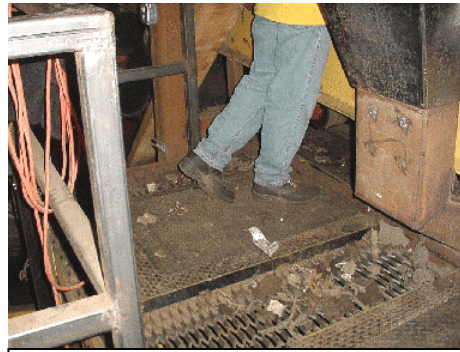
New Adjustable Work Platform.
