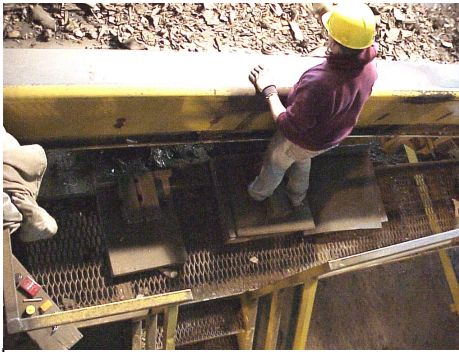
Original conveyor section and platform.
